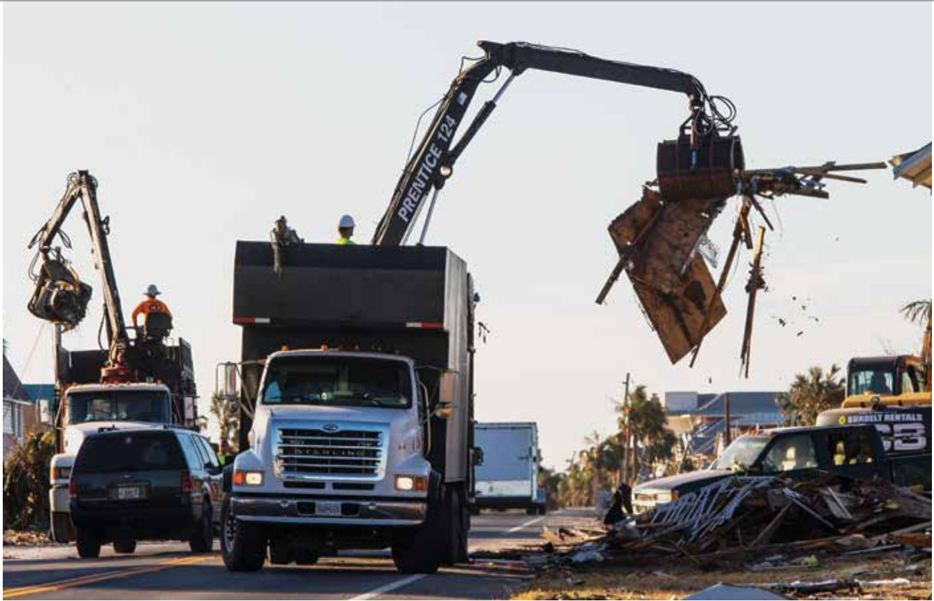
RECOVERY IS STILL UNDERWAY in the storm-ravaged Florida Panhandle, which saw entire communities erased from the landscape. Civil and environmental engineers at the FAMU-FSU College of Engineering are studying evacuation, resilience, recovery and sheltering practices and outcomes in the state to help inform disaster policy and planning nationwide. This photo shows initial disaster cleanup from Hurricane Michael on October 16, 2018 in Mexico Beach, Florida. Many students, faculty and staff volunteers helped clean up.
